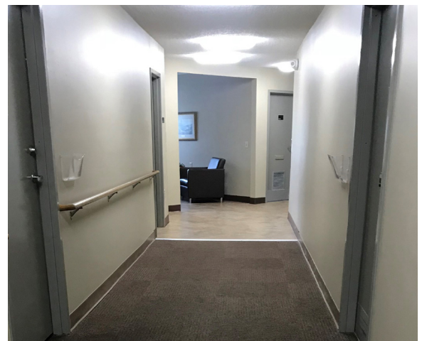
New hallway railings in the main building.
