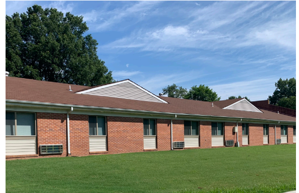
Inefficient centralized HVAC systems were replaced with efficient PTAC units located in each apartment.
