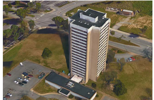
Aerial view of 18-story River View Tower prior to moderate rehabilitation.
