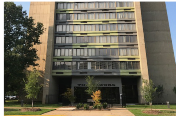
View of River View Tower front entrance after completion of moderate rehabilitation.
