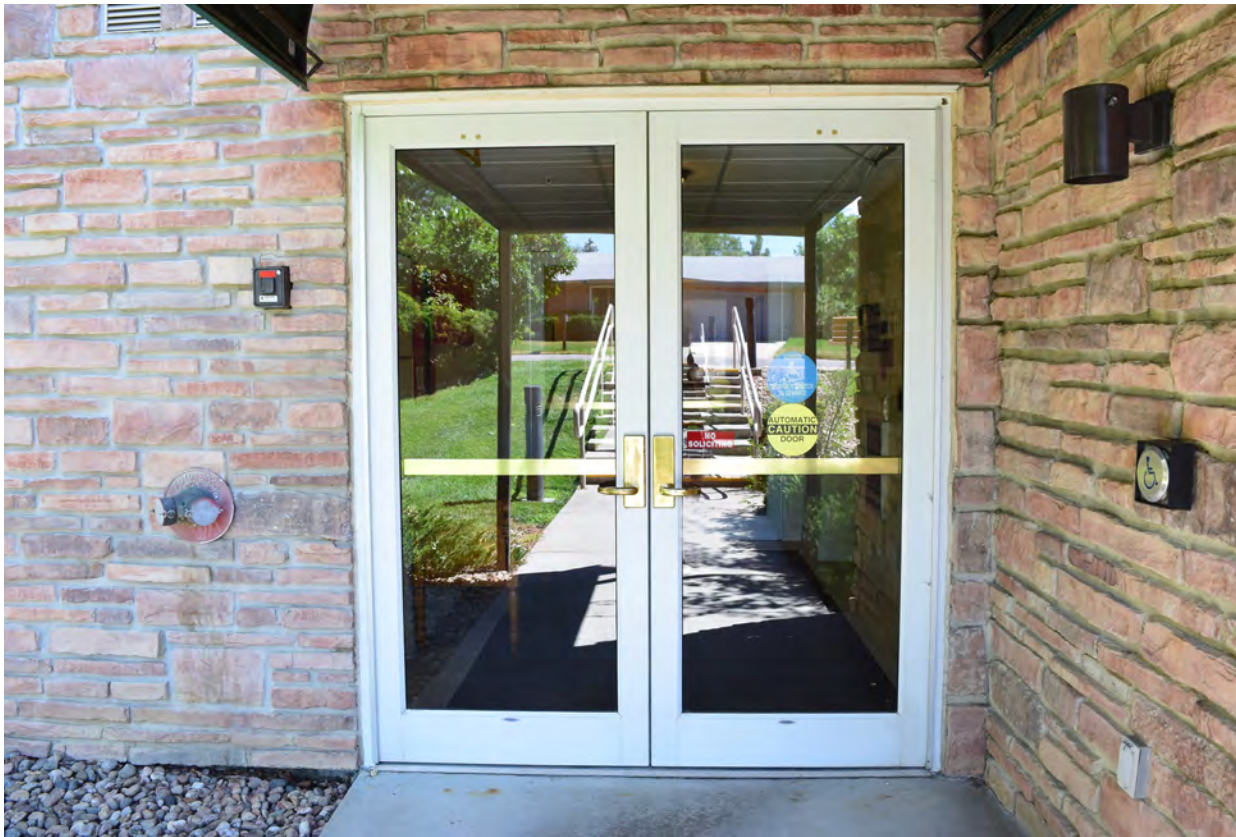
Main entry doors can be renovated with an automatic door system and wall mounted actuator.
