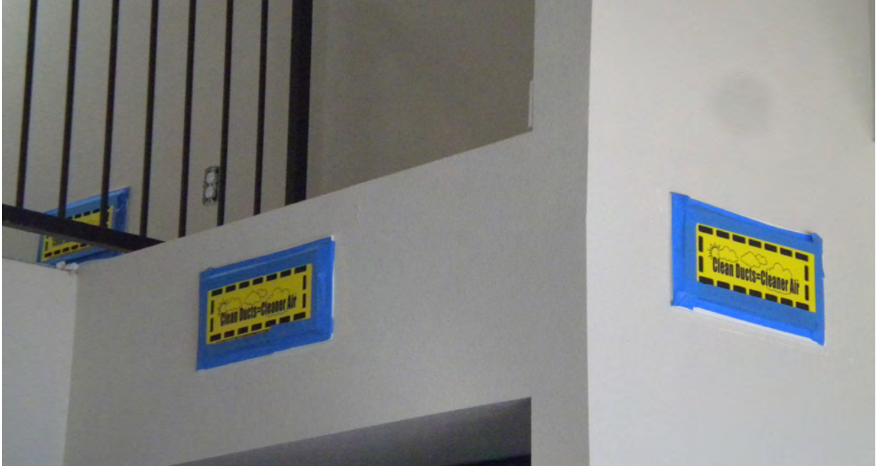
Protect ductwork from dust and debris during construction.
