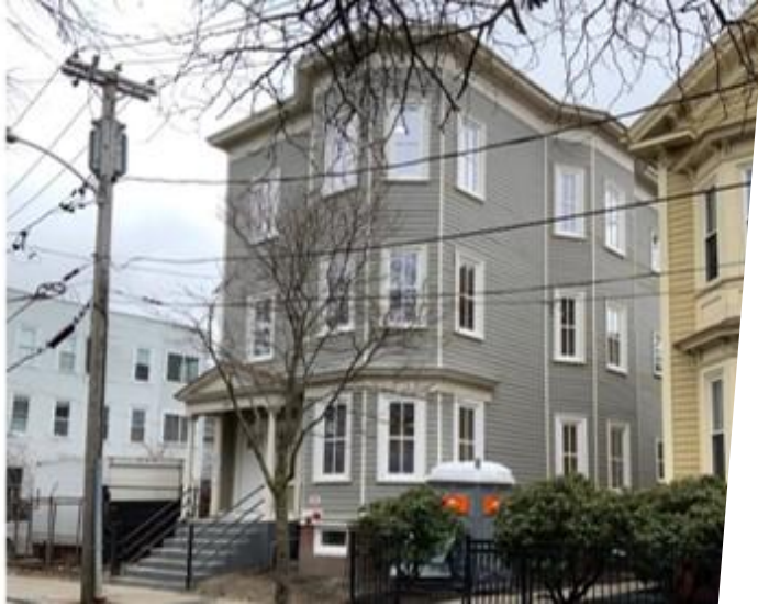
171-173 Columbia St. Is a green and affordable triple-decker rehabilitated from a fire in 2020. (Courtesy of HRI)
